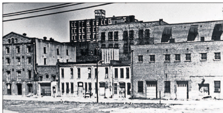
The Cotton Exchange in 1973, a year before restoration work began. [CONTRIBUTED PHOTO]
