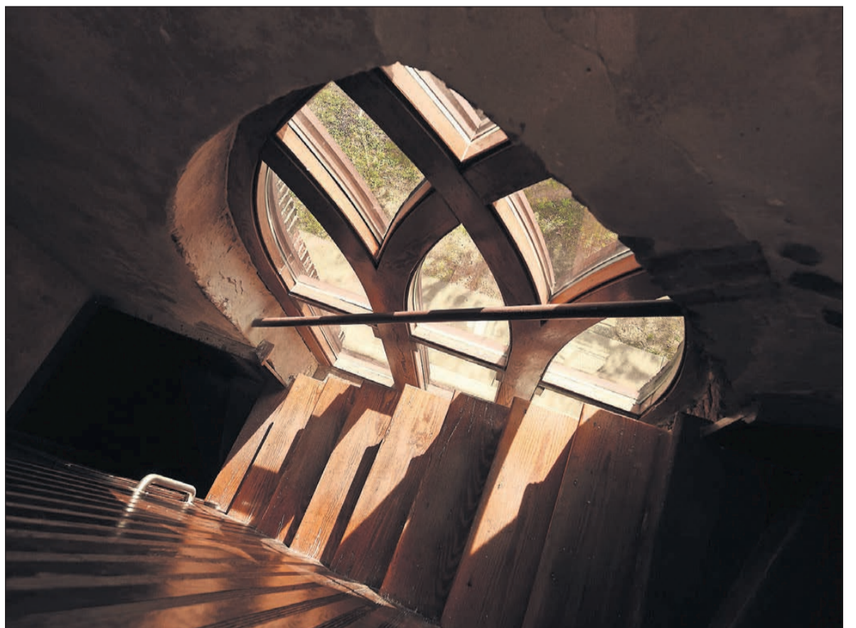
Before its restoration, bracing had to be added to the St. Andrew's Church building to keep the walls from collapsing.
