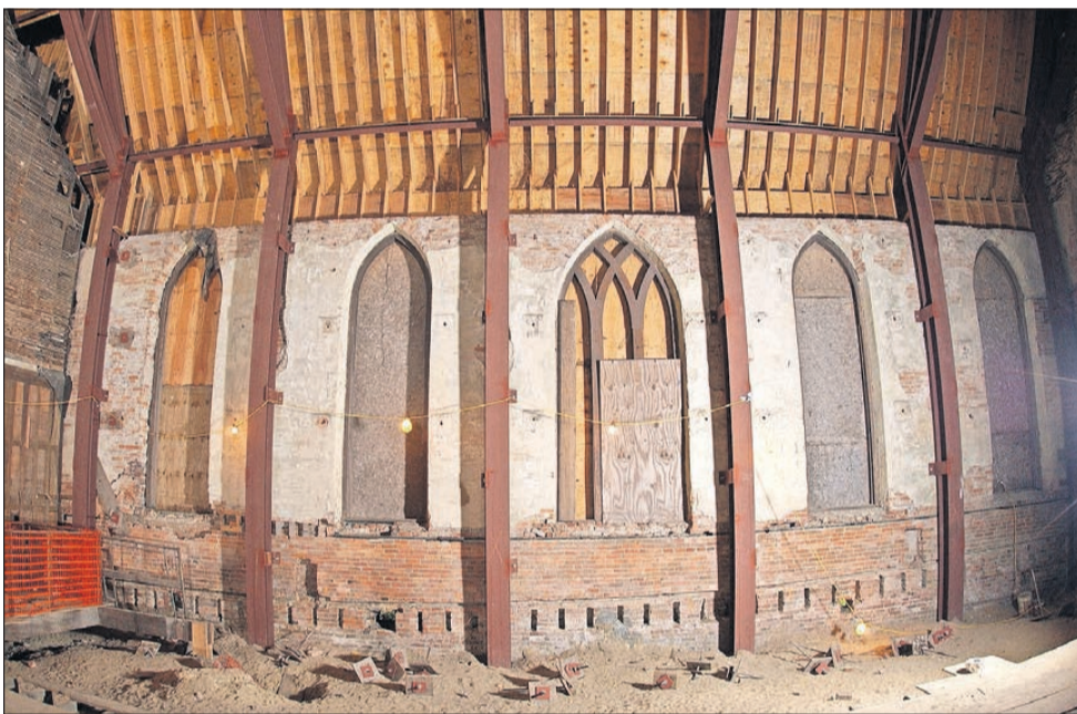
Before its restoration, bracing had to be added to the St. Andrew's Church building to keep the walls from collapsing.
