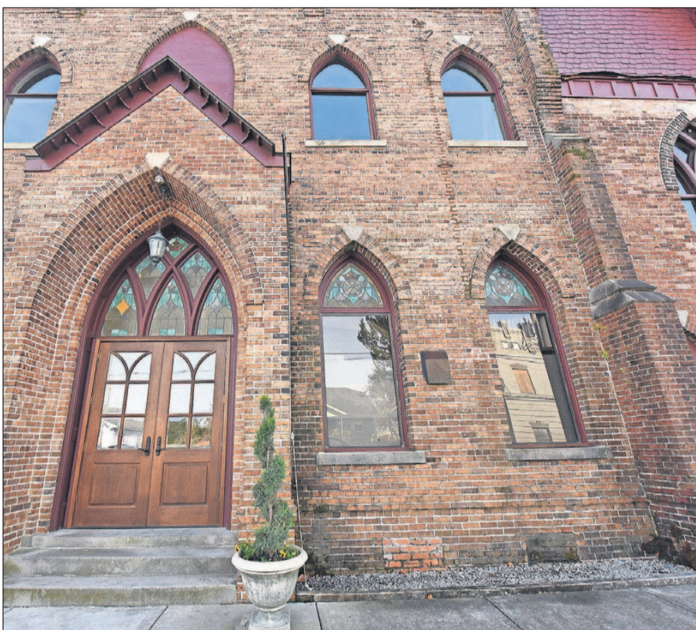
St. Andrew's Presbyterian Church opened its doors in 1888. Over the years, the structure fell into disrepair. Today it is the Brooklyn Arts Center and serves as a symbol of the revitalization of the North Fourth Street and Brooklyn areas. [STARNEWS FILE]
